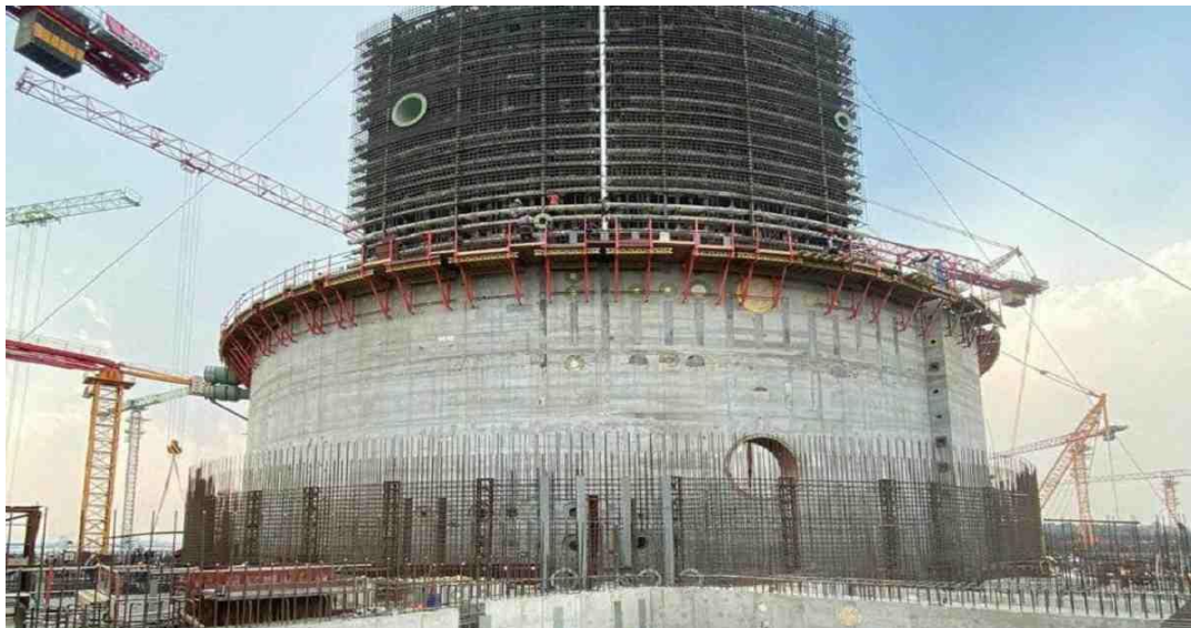
Figure: 2. A 10 m high section of turbine building, RAPP-5&6 built with SCC
