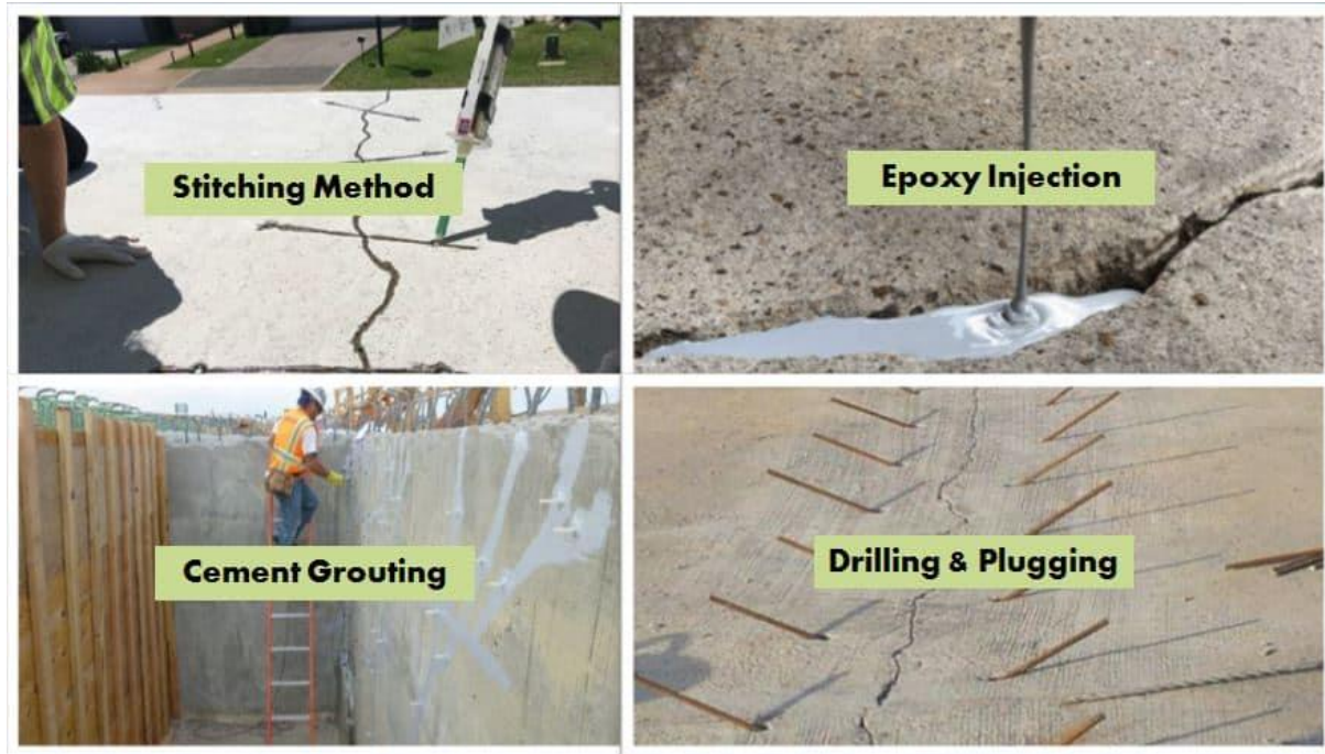
Fig :- Different Repairing Method
