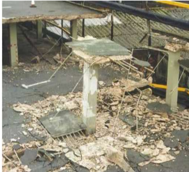
Figure-2 Typical punching shear failure [3].
