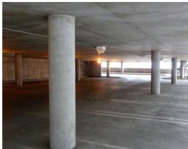
Figurer-1 Flat plate concrete construction [2].
