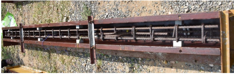
Fig. 1 Steel Bars Grill in Beam Mould
