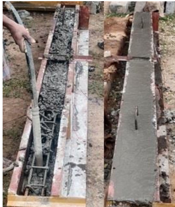
Fig. 3 Casting of Beam
