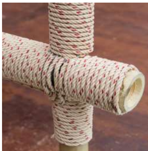
Fig 4. Bamboo joint used ordinary fiber “Nylon” rope by the region of their bond
