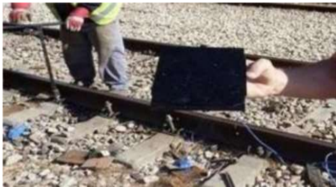
Fig.2.5 Installing Piezo IPEG Pads
