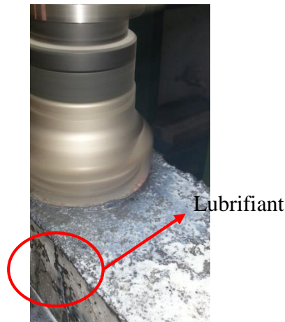
Figure9. Surfacing of new concrete with lubrication
