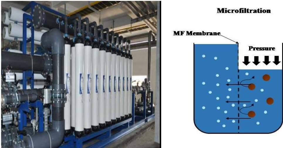
Figure 9, 10: Ultrafiltration and Microfiltration for Wastewater Recycling
