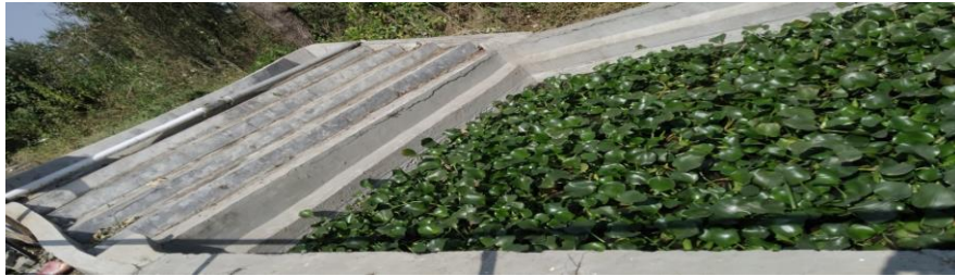
Figure 1: Treatment of wastewater
